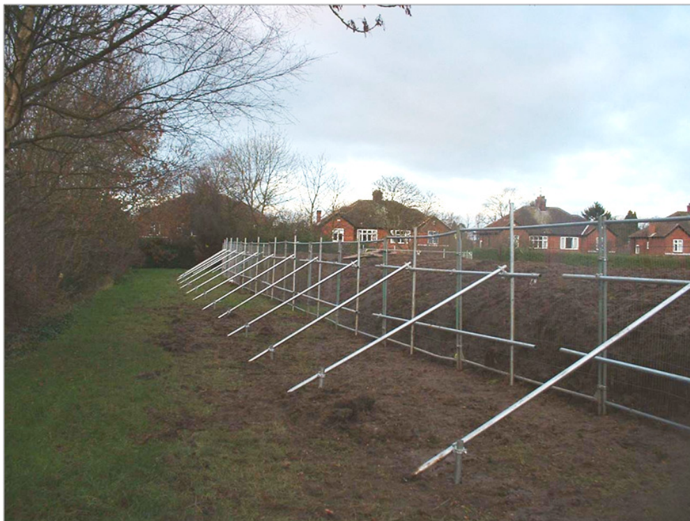
Figure 3 - Example of a barrier erected on a site
